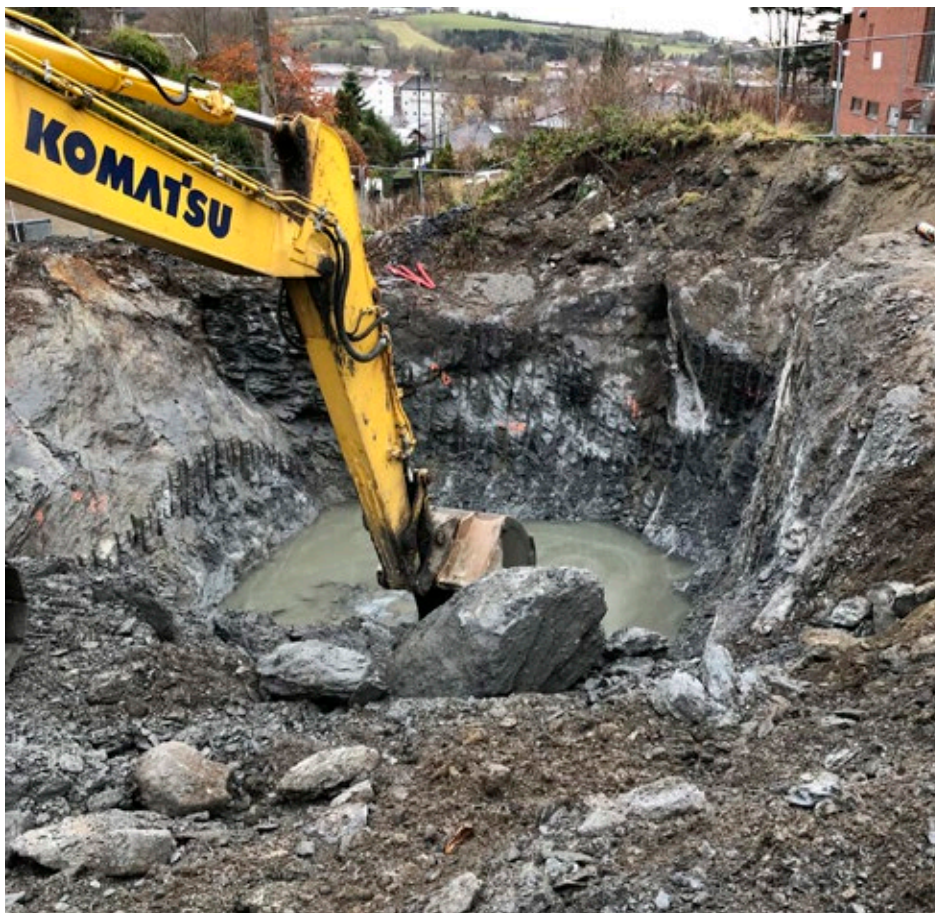
Excavation of the fell for the stage in Hinna, Norway.
